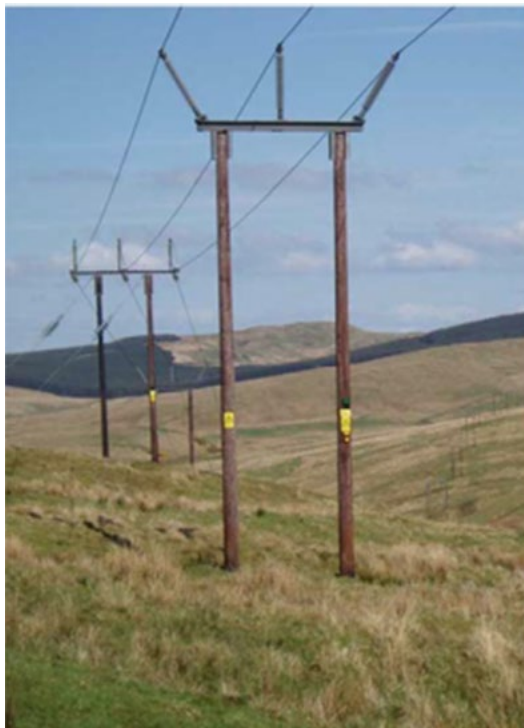
Plate 1.1 – Typical trident pole configuration
