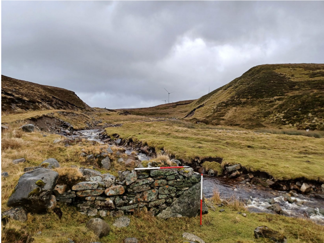
Plate 7.3– Photo of Building at River E (HA4). The pictured wall is the only surviving element of the building seen. February 3 rd , 2022.
