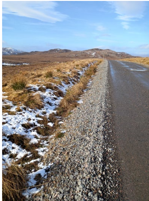
Photograph 2-B – Drain 2, taken at NGR 255199 813650
