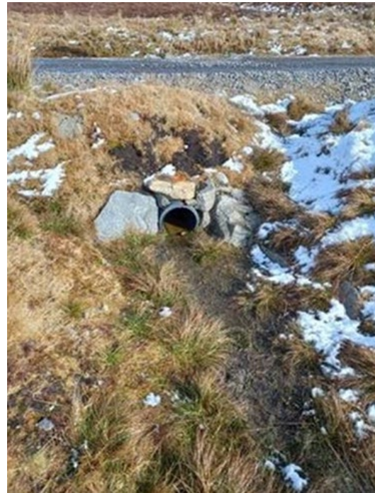
Photograph 1-B – Culvert B, taken at NGR NH 255202 813641.
