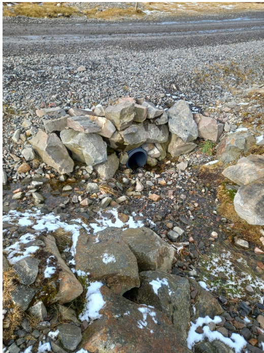
Photograph 1-A – Culvert A, taken at NGR NH 254736 813965.
