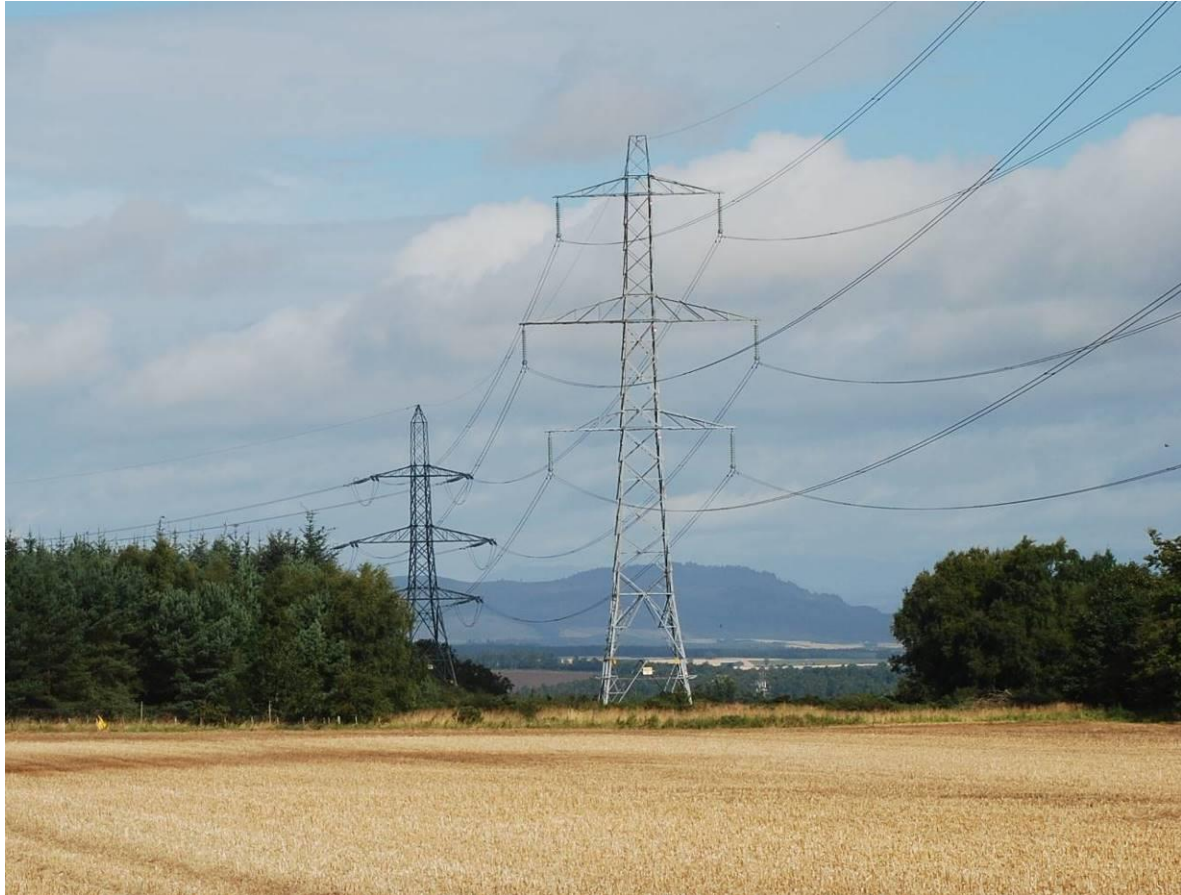
Typical L8 line tower and (partly behind trees) angle tower
