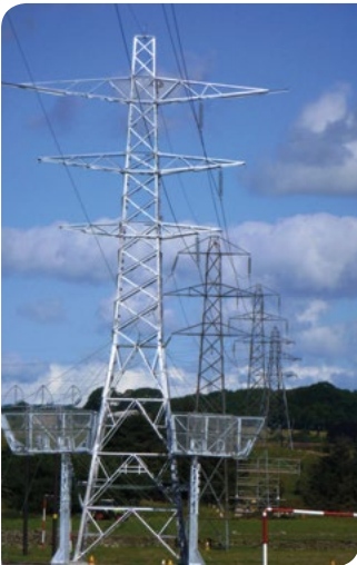
Aberdeen WPR bypass project (PTDYE451)
