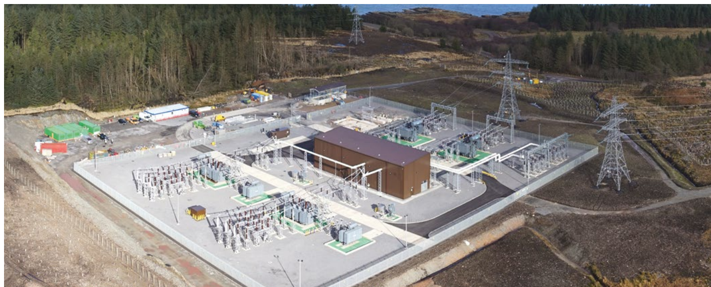
Crossaig Substation – this is an example of a Transmission substation in Kintyre
