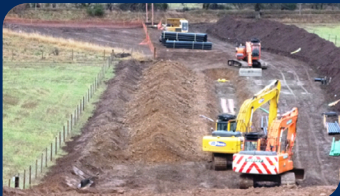
Construction of an Underground Cable trench
