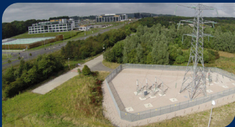
An example of a Sealing End Compound
