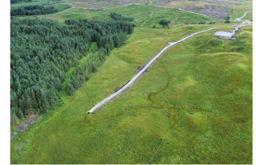
Final access track completion
