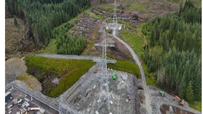
Towers 1 and 2 topped out at substation (Creag Dhubh to Dalmally side)
