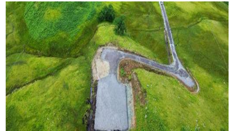
Access track completion
