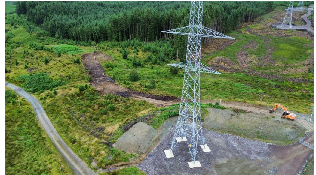
Underground works complete at Tower 33
