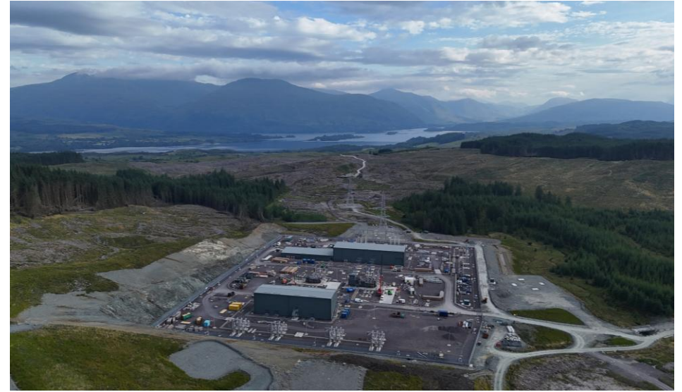
Creag Dhubh site overview — July 2026
