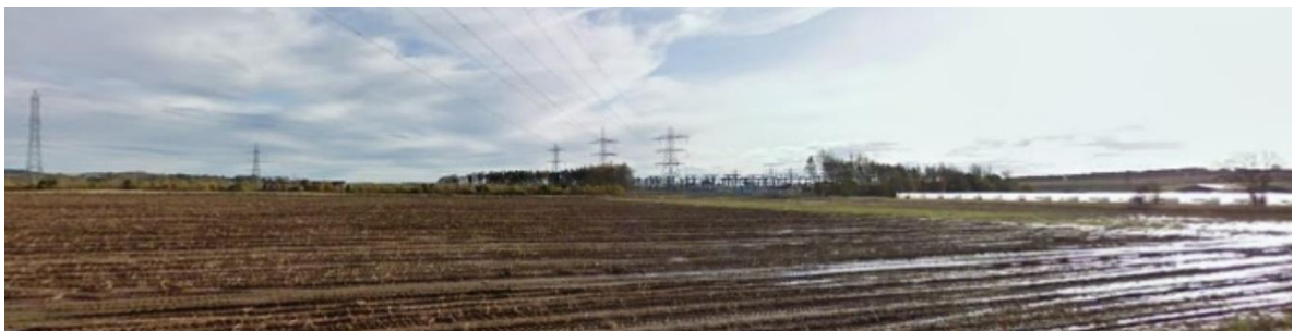
Photo 3: Tealing substation from minor road to the west of the substation, just north of Fithie Burn [Source: Google Streetview]
