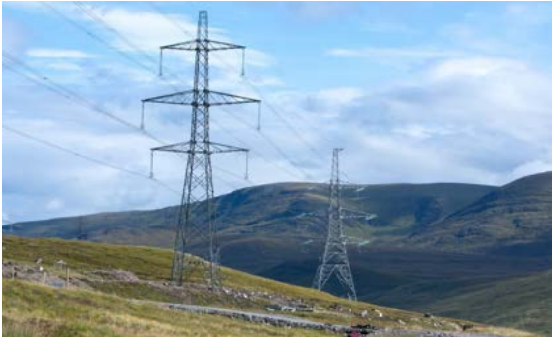
Plate 2.1 – Typical SSE400 steel lattice tower design
