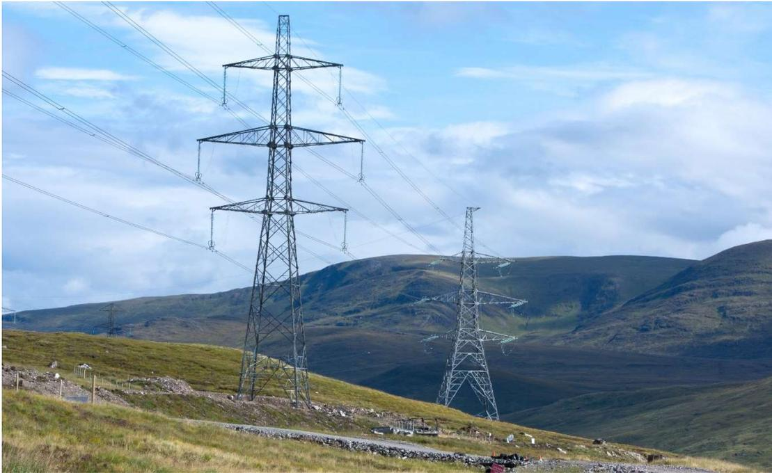
Plate 2.2 – Typical SSE400 steel lattice tower design (Schematic)
