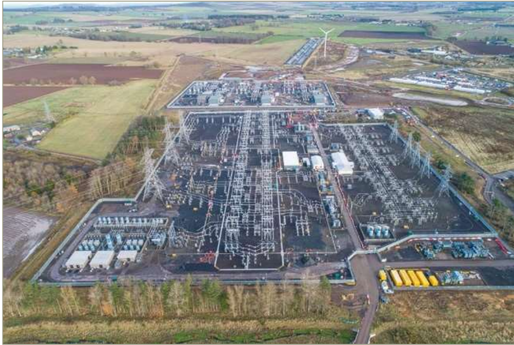
Plate 2.1 - Aerial Photograph of the Existing Tealing Substation
