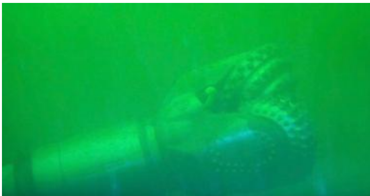
HDD drill emerging on seabed
