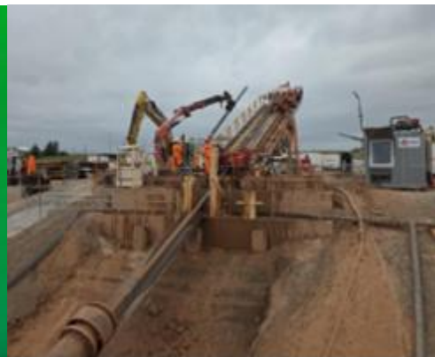
HDD landfall drill rig in operation
