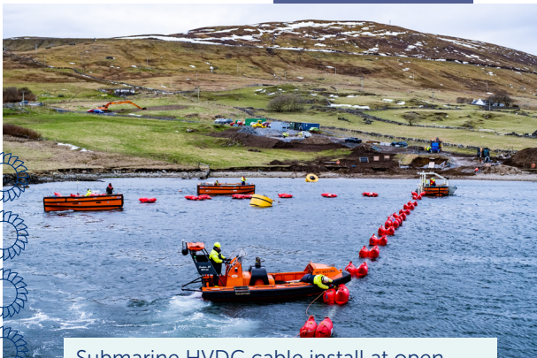
Submarine HVDC cable install at open cut trench landfall using a float-in method
