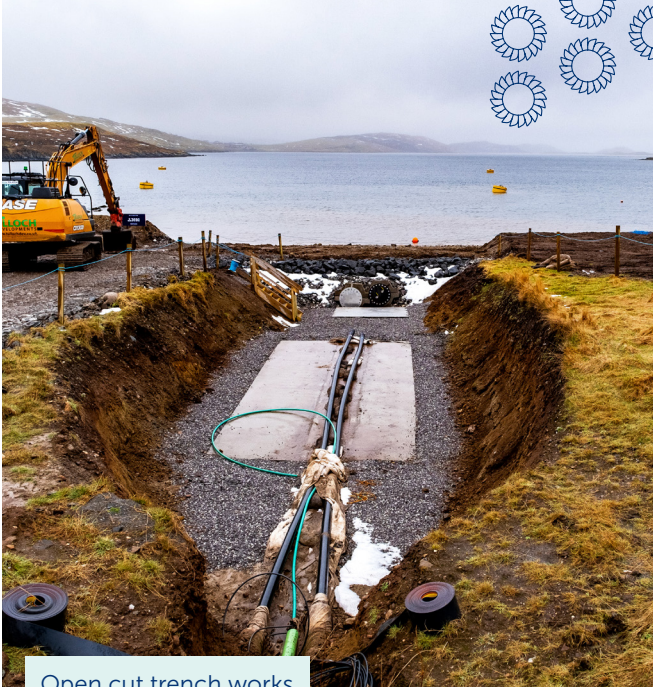
Open cut trench works
