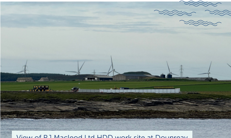
View of RJ Macleod Ltd HDD work site at Dounreay
