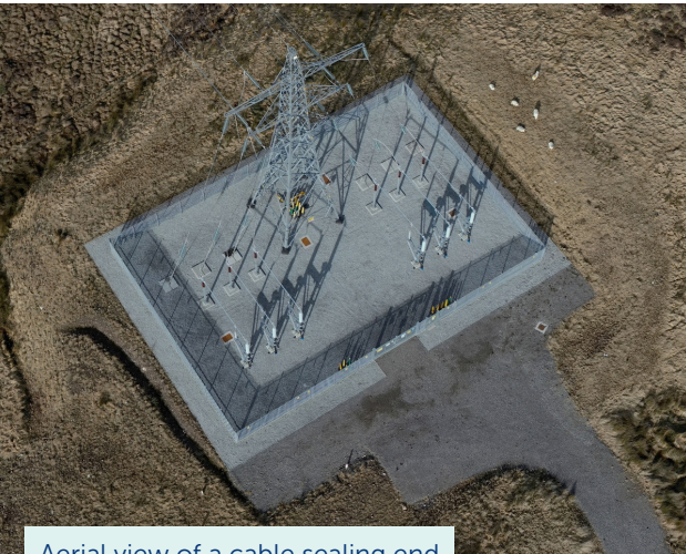
Aerial view of a cable sealing end
