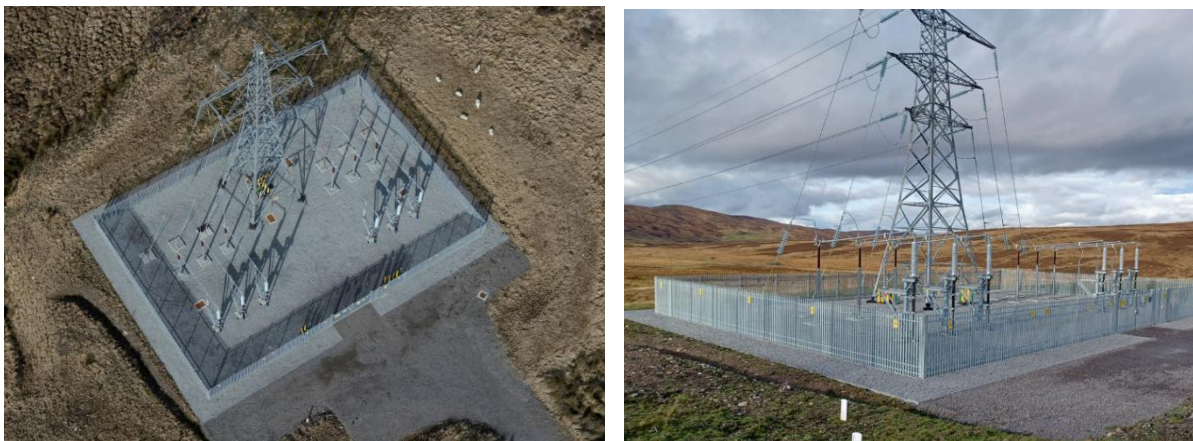
Figure 2-2 Typical cable sealing end compound
