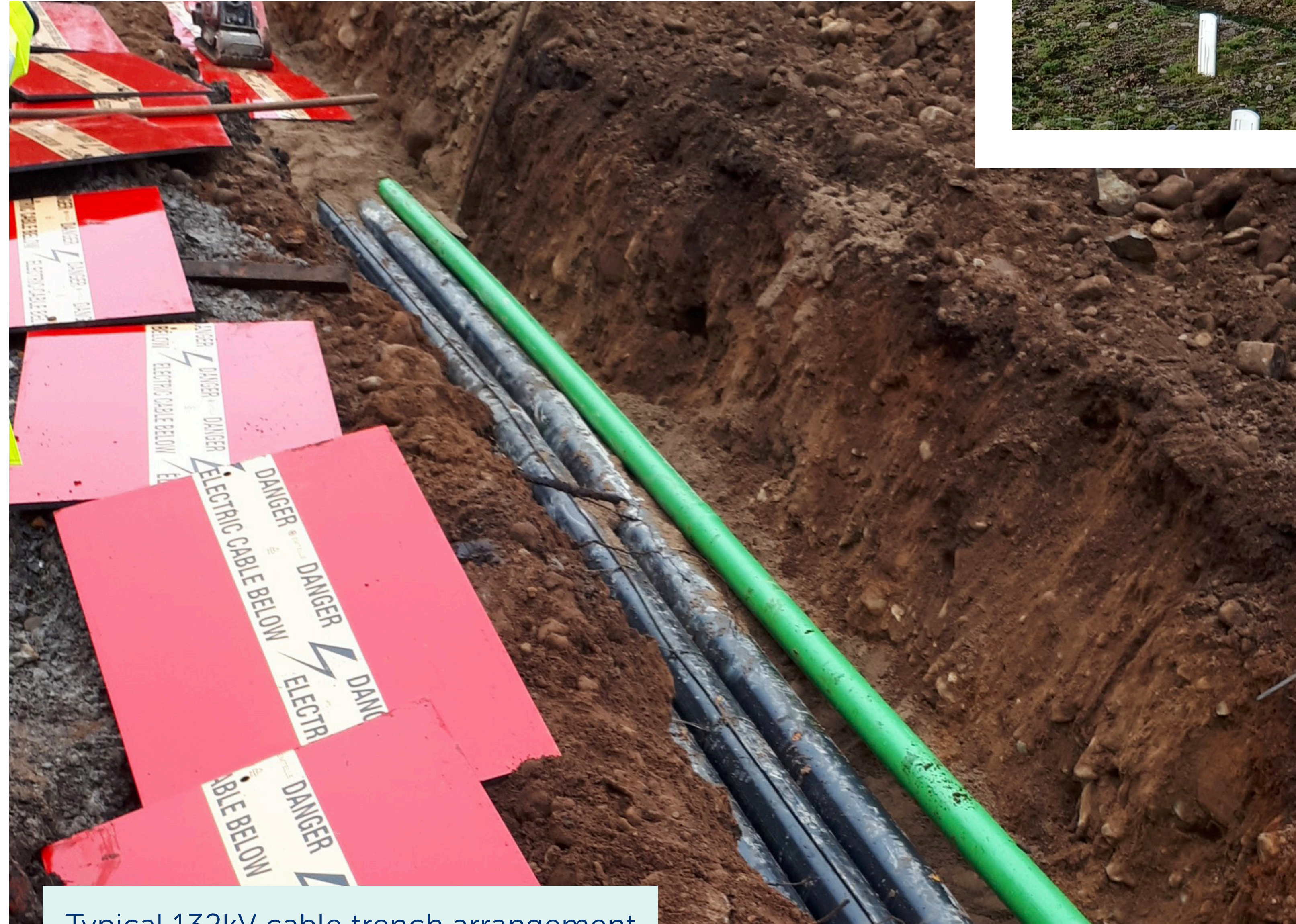
Typical 132kV cable trench arrangement
