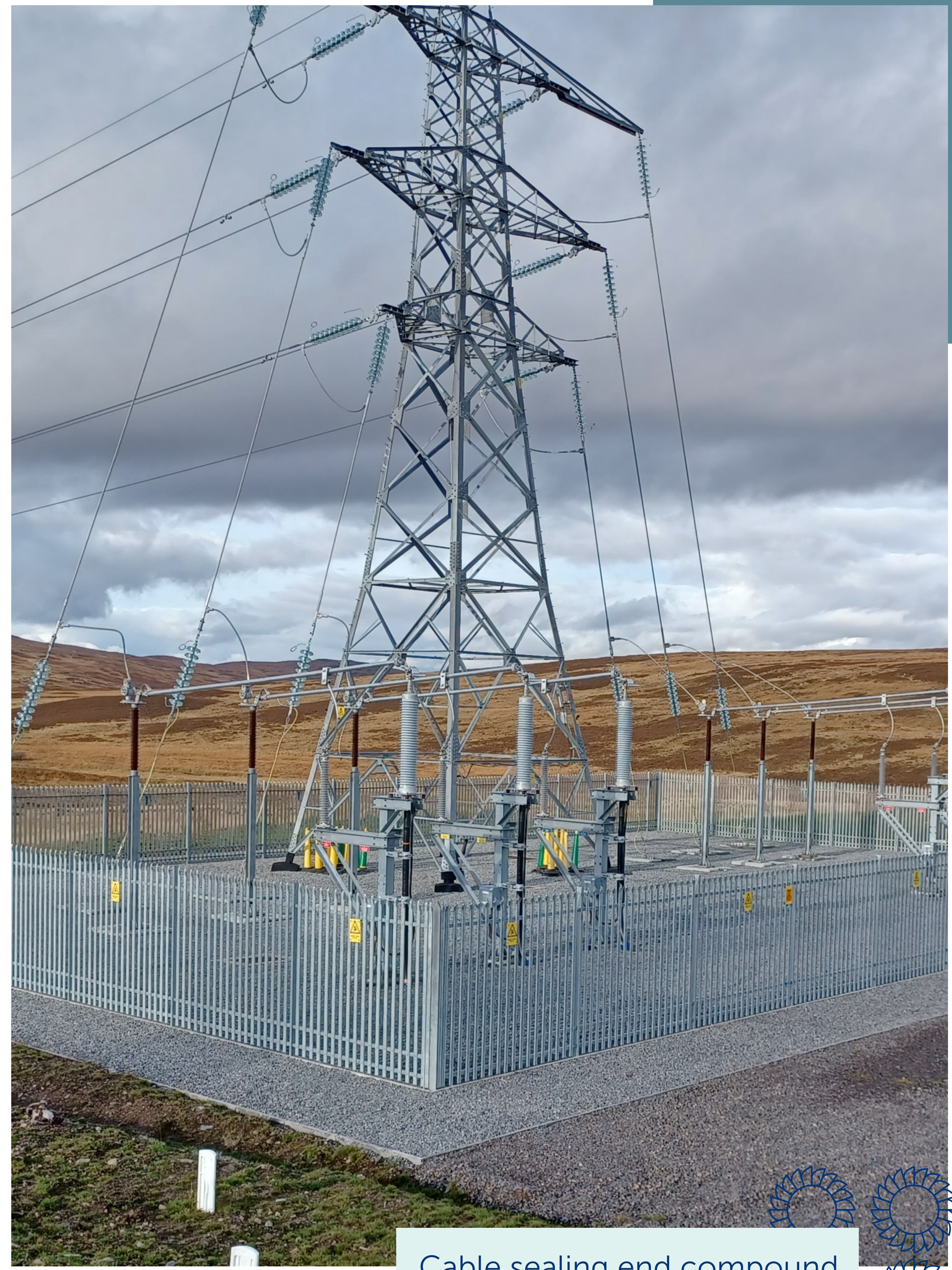
Cable sealing end compound
