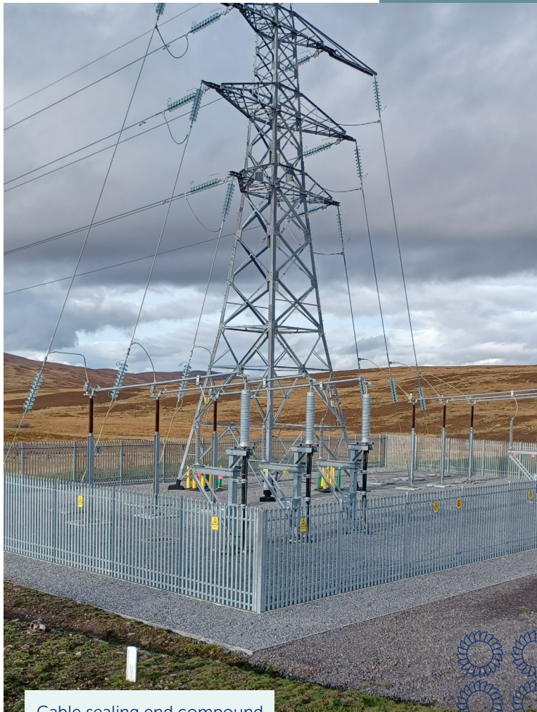
Cable sealing end compound
