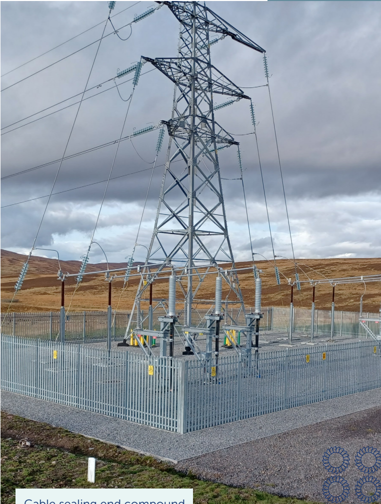
Cable sealing end compound
