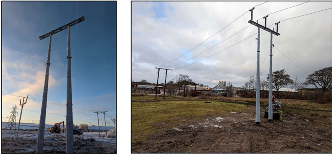
Plate 2.1: Example Steel Trident H Poles
