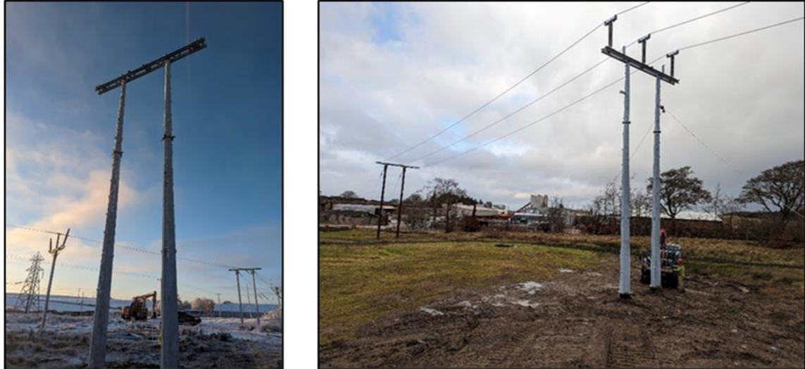
Plate 3.1: Example Steel Trident H Poles
