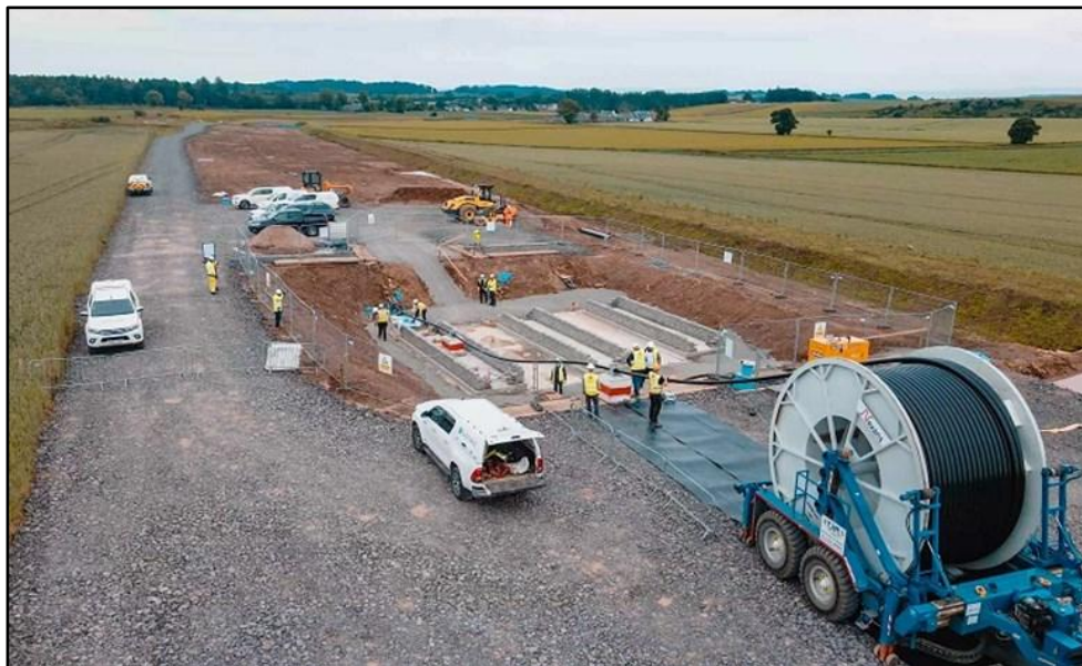
Plate 3.2: Photograph of Underground Cable Installation
