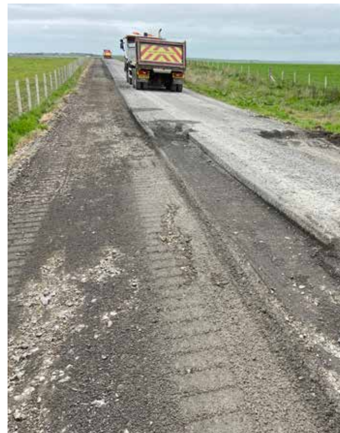
Haul road being removed
