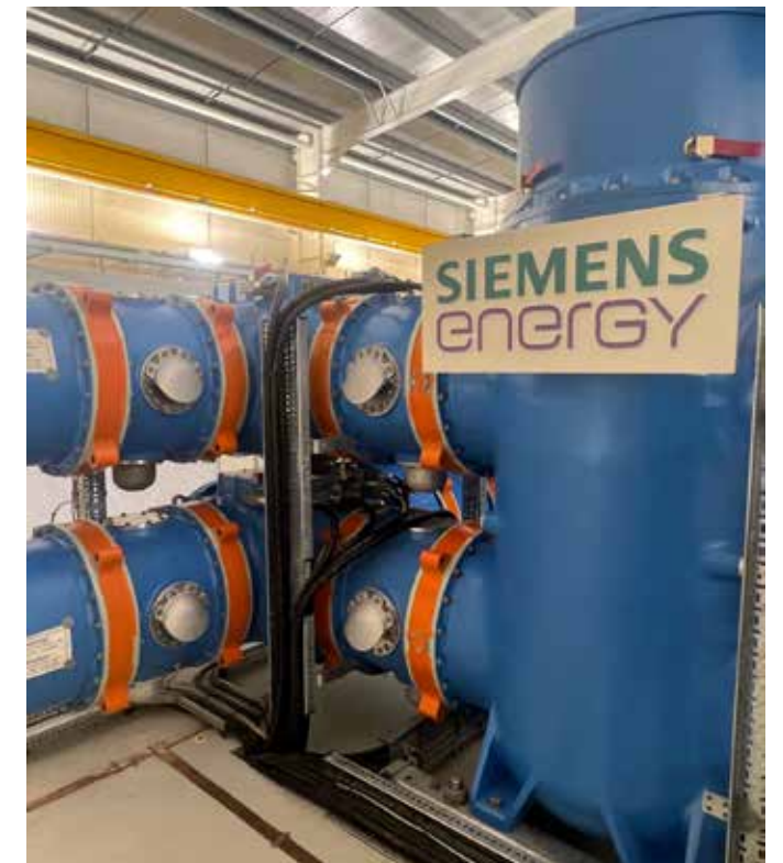
Painting gas tight barriers
