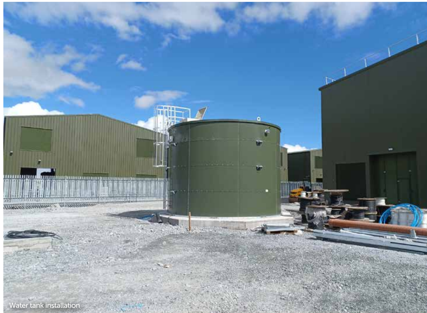
Landscaping works ongoing and water tank installation
