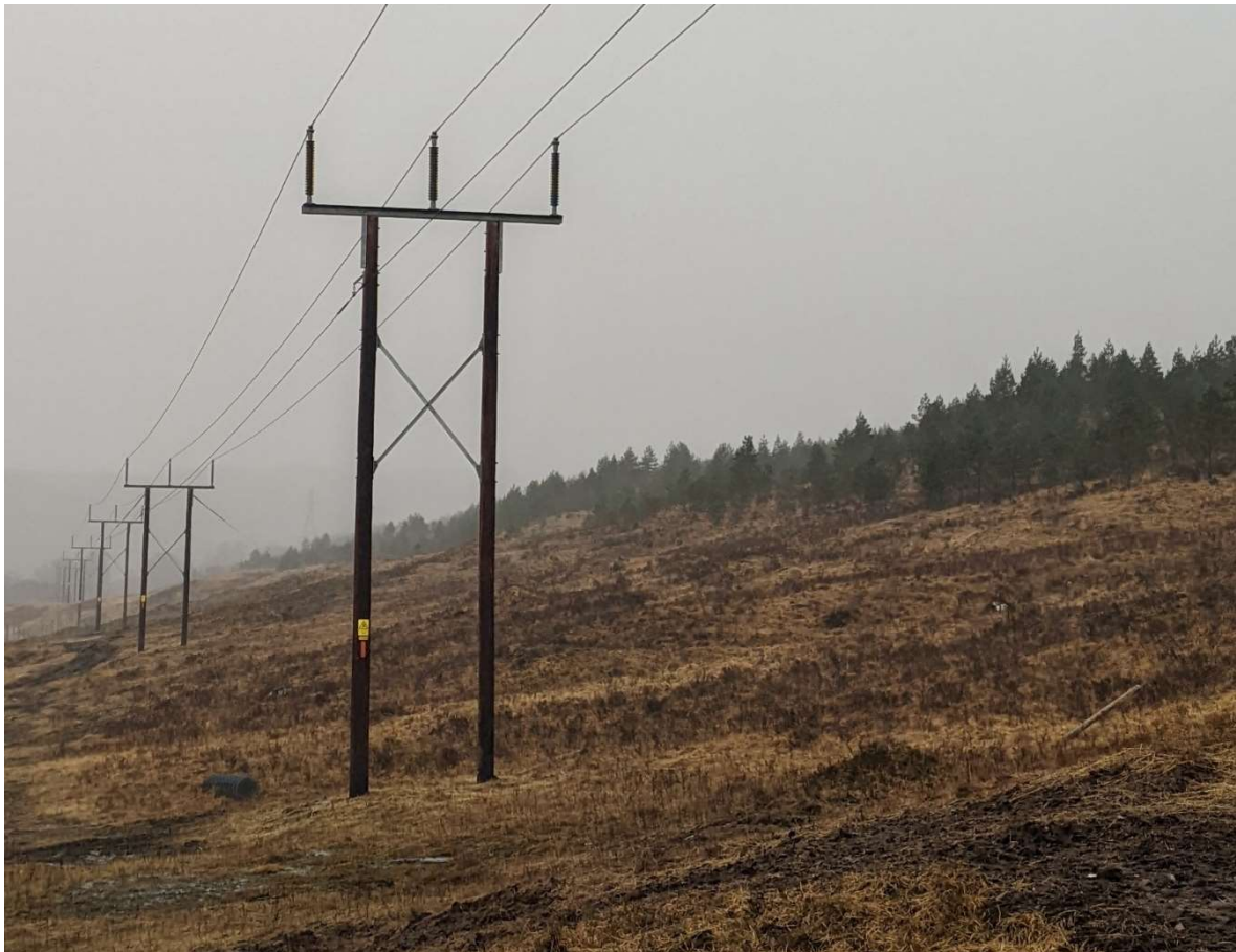
Plate 2.1: Trident wood pole design
