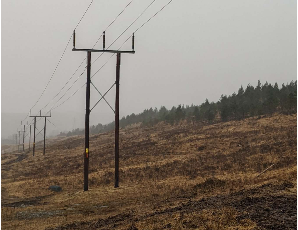
Plate 1.1 Typical Trident wood pole design
