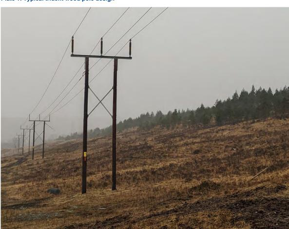
Plate 1: Typical trident wood pole design
