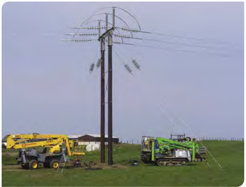
Above is a typical example of an angle wood pole which requires additional stays. Please note the stays will not be on the non-angle poles.
