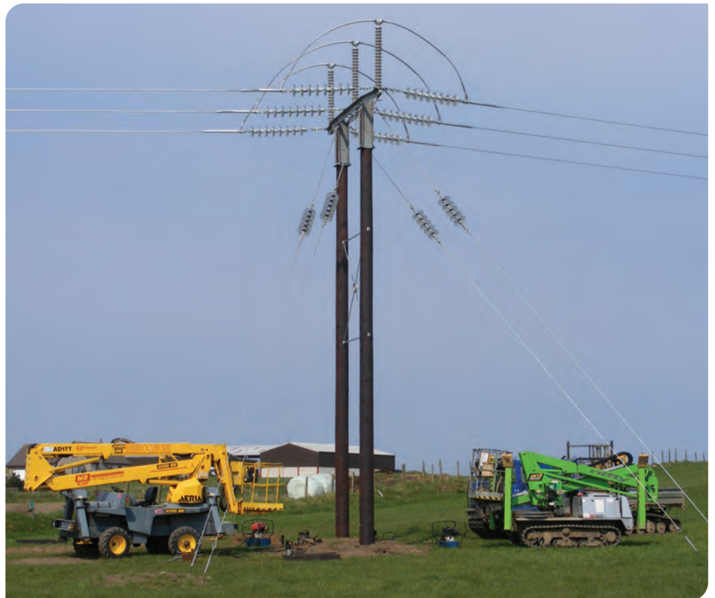
Above is a typical example of an angle wood pole which requires additional stays. Please note the stays will not be on the non-angle poles.
