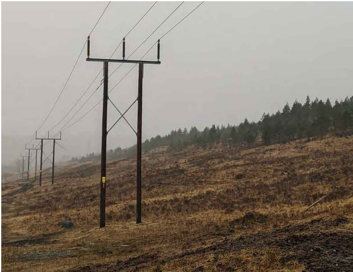
Plate 2.1: Trident wood pole design
