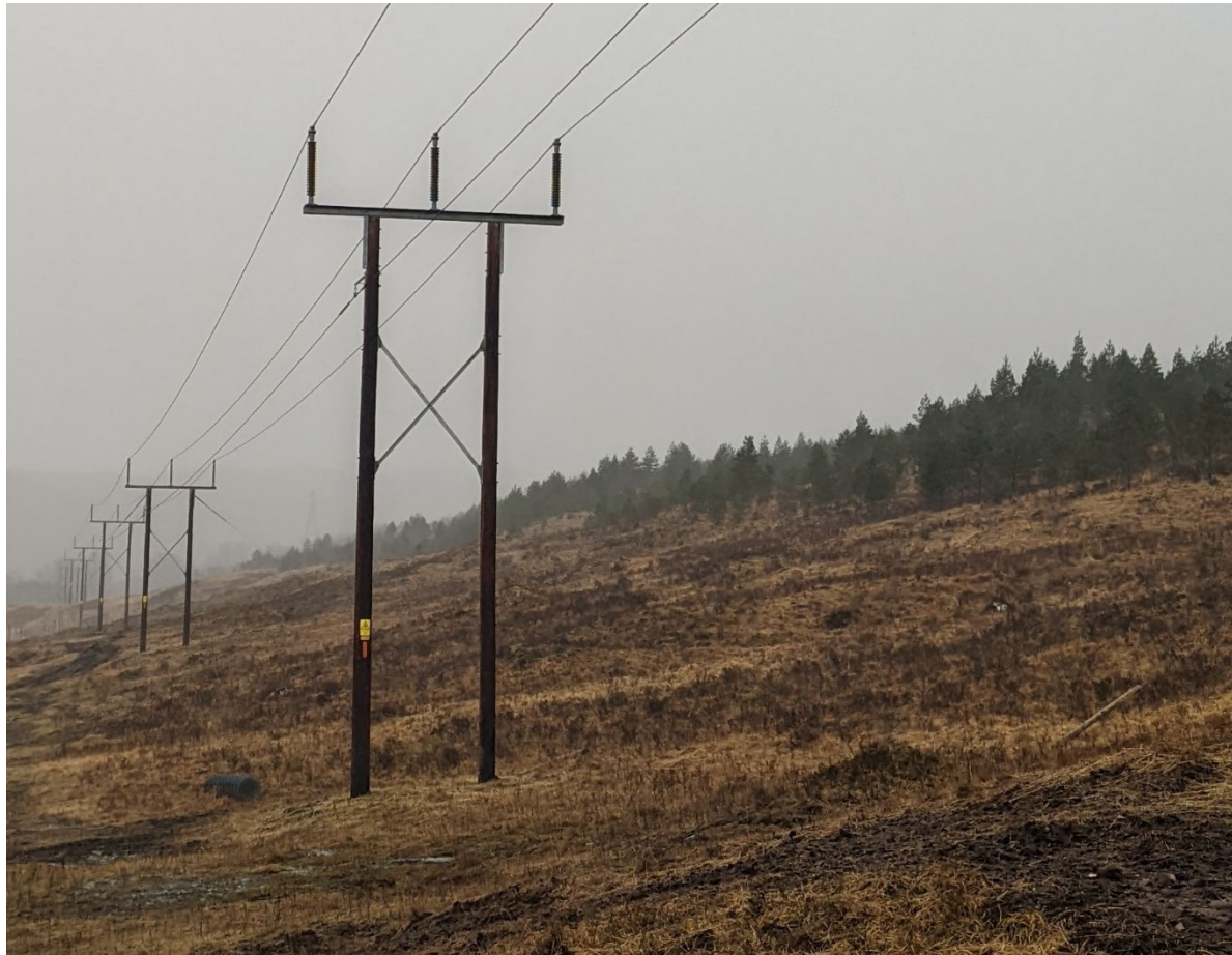
Plate 2.1: Typical trident H pole design
