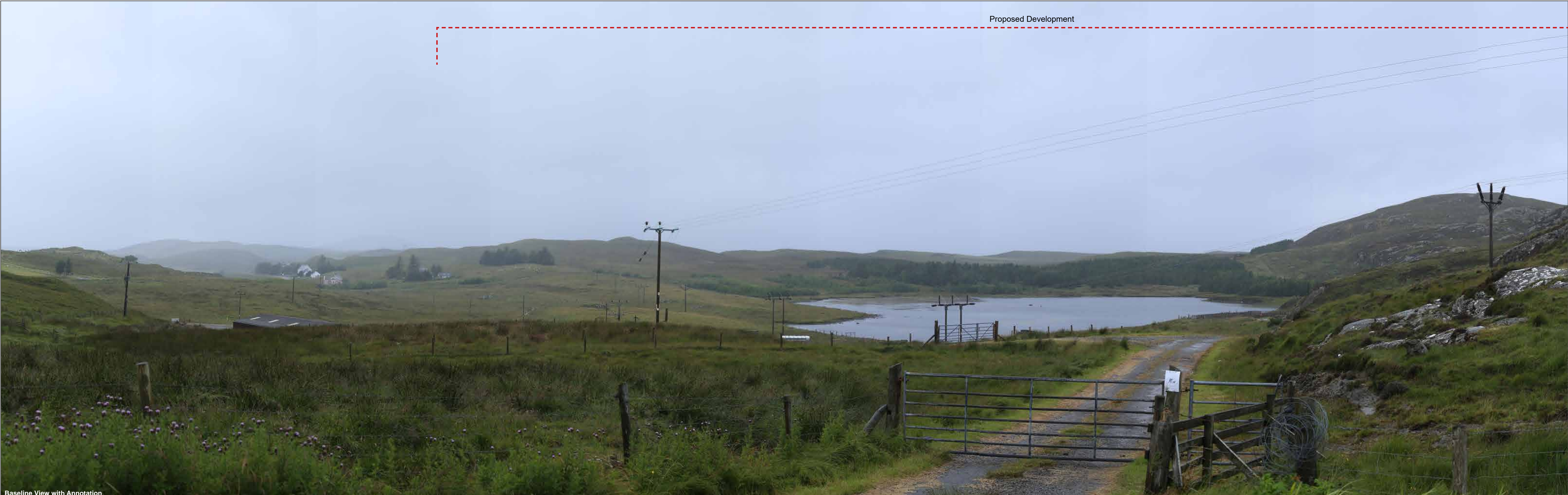
Baseline View with Annotation Figure 6.18e VP12: Laxay Harris to Stornoway 132 kV Overhead Line Replacement
