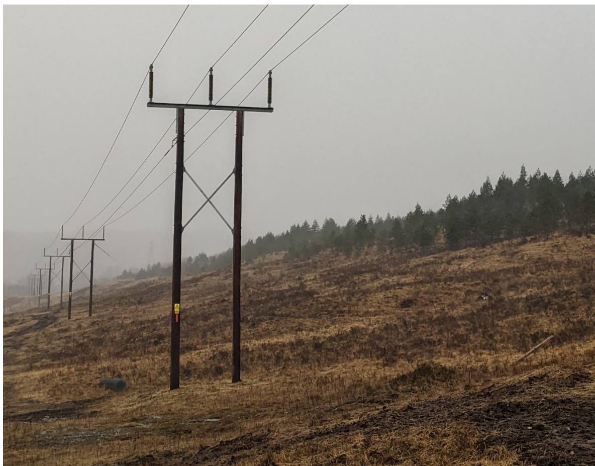
Plate 1: Trident wood pole design
