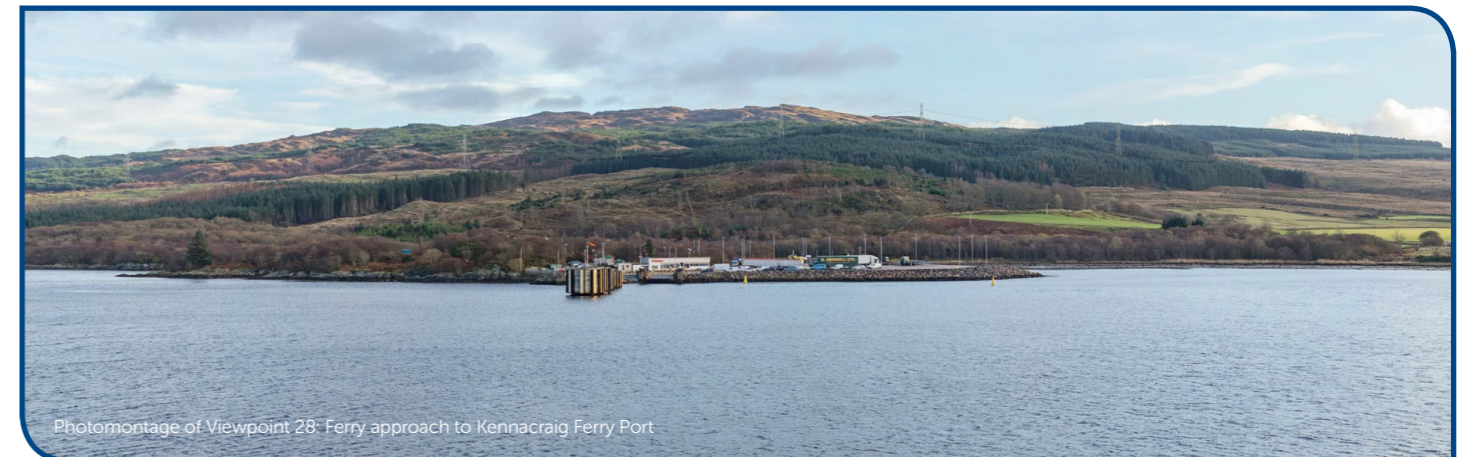
Wireline of Viewpoint 28: Ferry approach to Kennacraig Ferry Port
