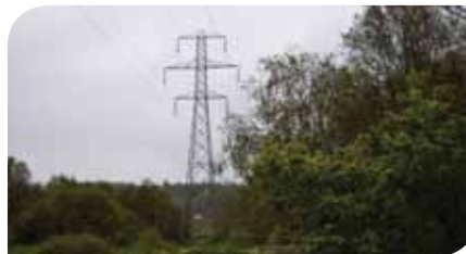
Existing PL16 Suspension Tower
