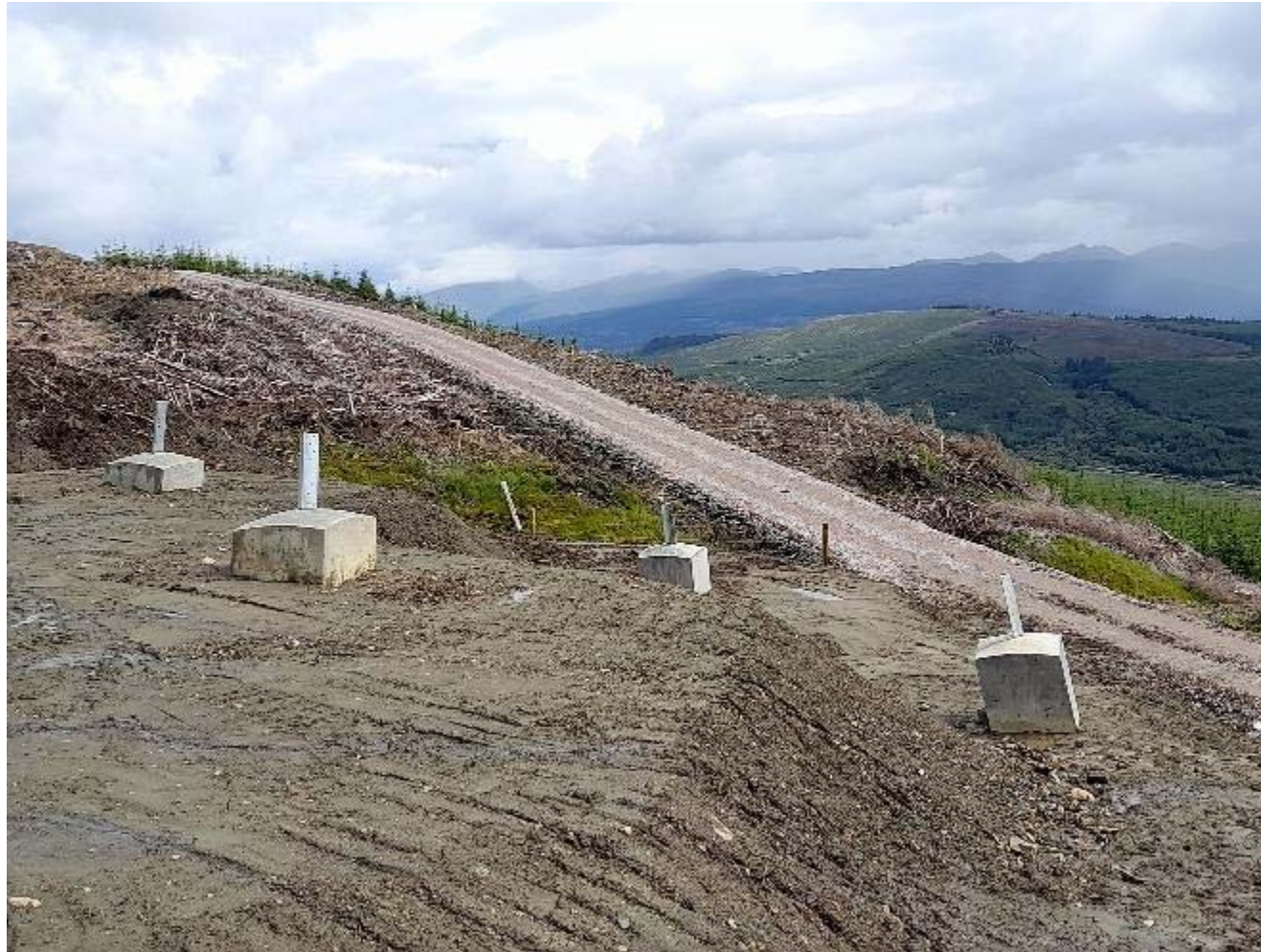
Tower 58 conventional foundation
