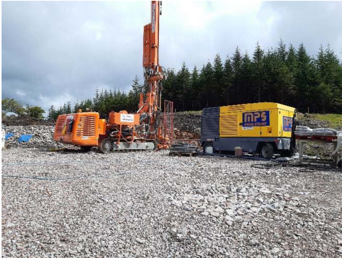
Tower 13R Piling
