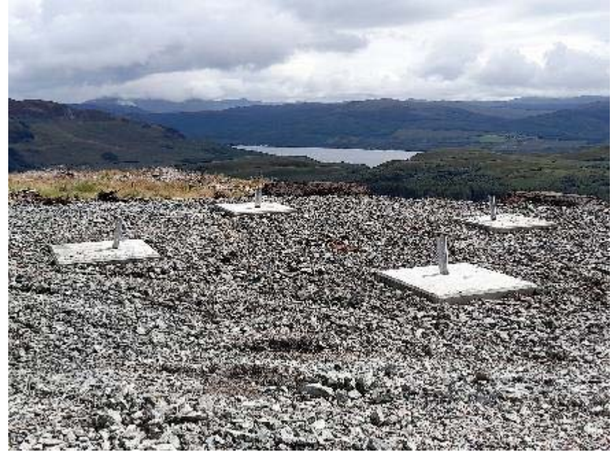
Tower 63 pile cap
