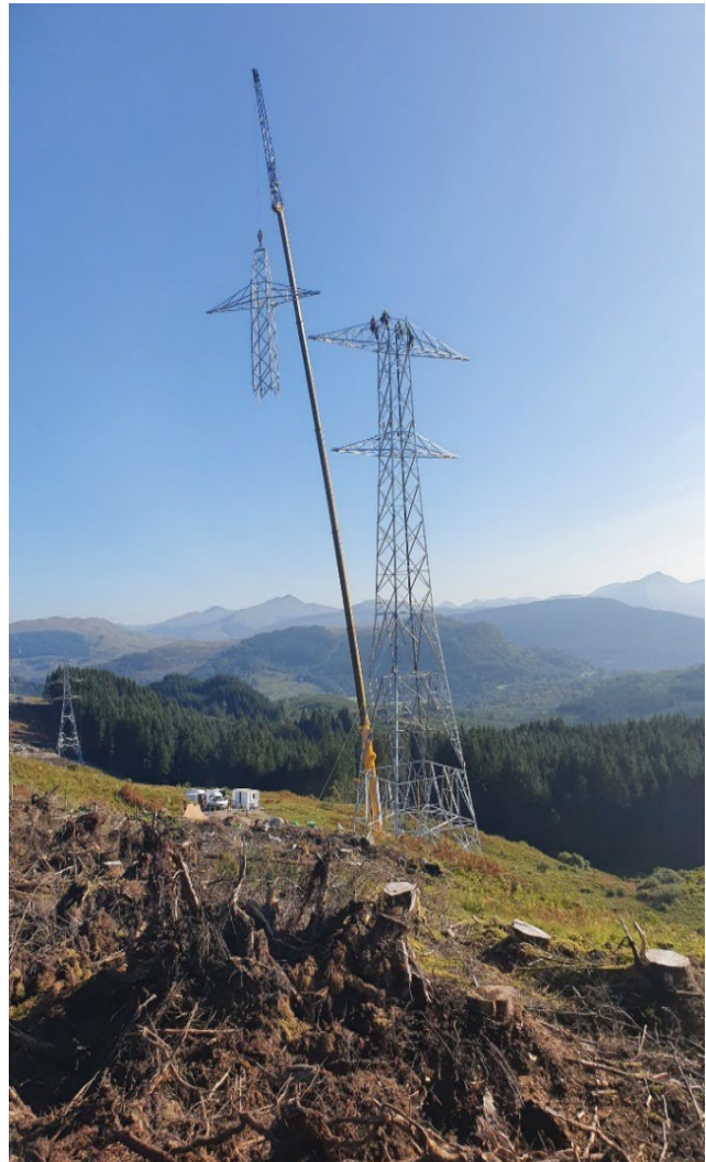
Representative Tower Construction
