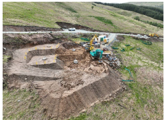
Representative Tower Foundation Construction
