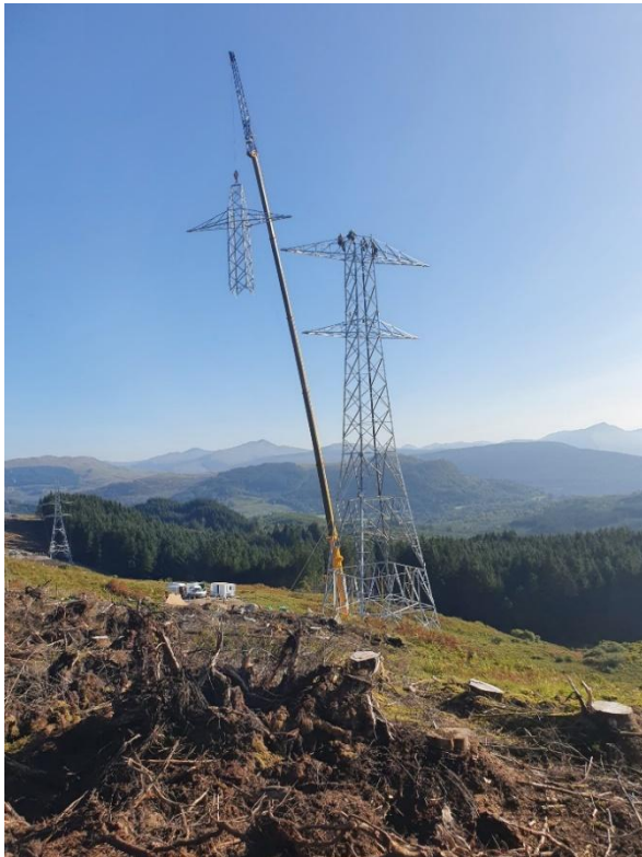
Plate 3.3: Illustrative Image of Tower Construction
