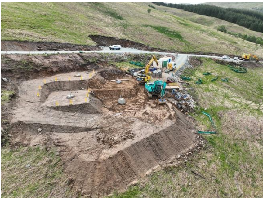
Plate 3.1: Illustrative Image of Tower Foundation Construction
