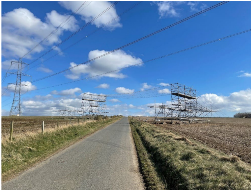
Plate 3.5: Illustrative Image of Temporary Construction Scaffolds
