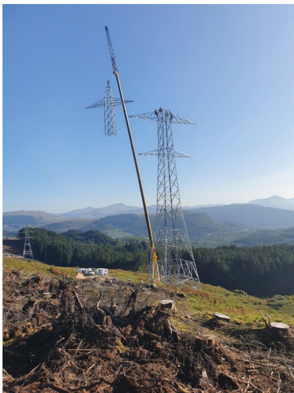
Plate 3.4: Illustrative Image of Tower Construction
