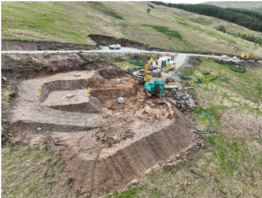
Plate 3.2: Illustrative Image of Tower Foundation Construction
