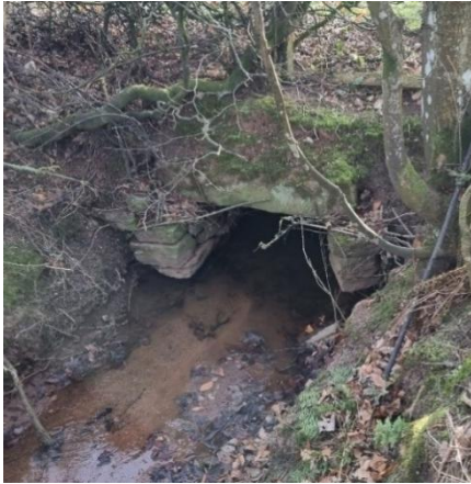
Stone Box Culvert
