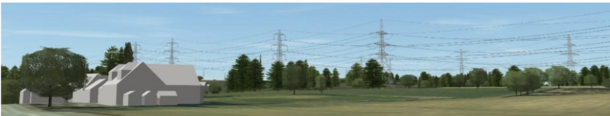
Section F – Entry to Kintore Substation looking Southwest
