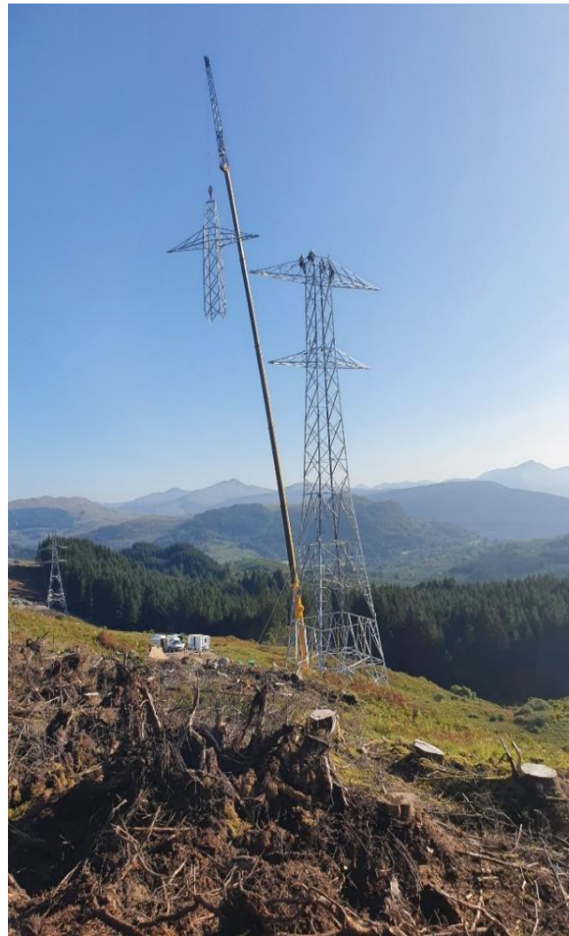
Representative Tower Construction
