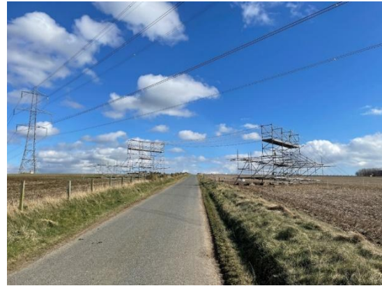
Representative Construction Scaffolds
