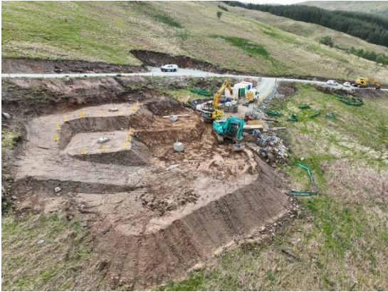
Representative Tower Foundation Construction
