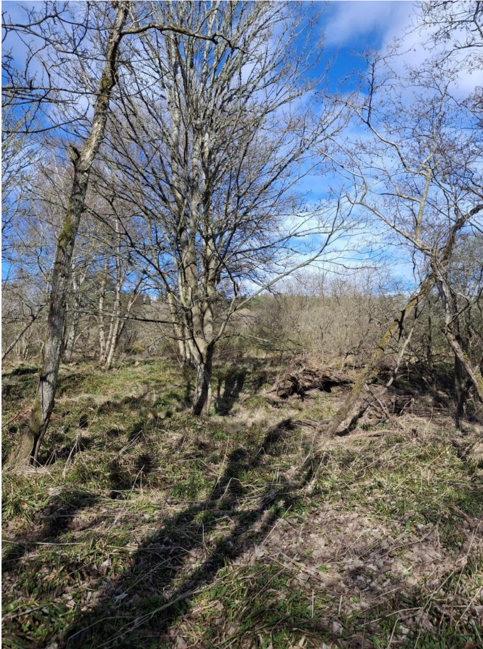
Plate 2: Looking north towards Tower N61
