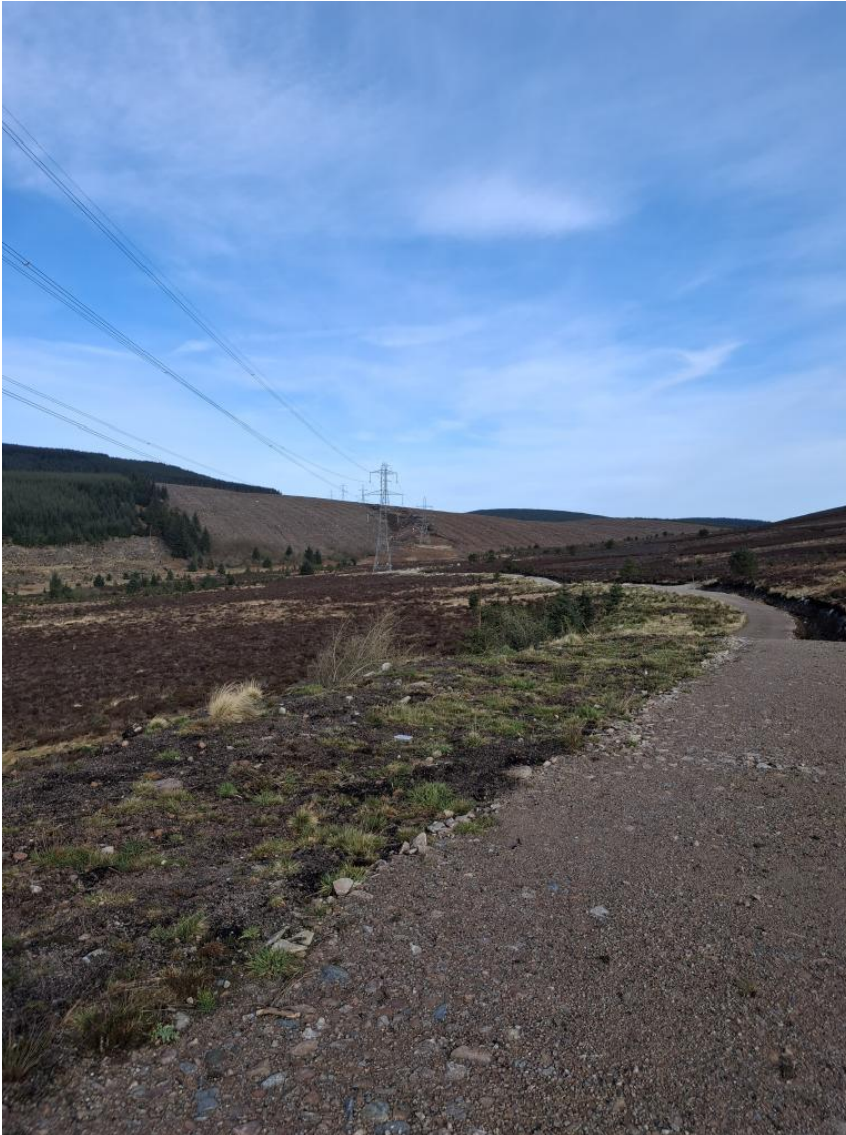
Plate 2: Looking north from tower N83
