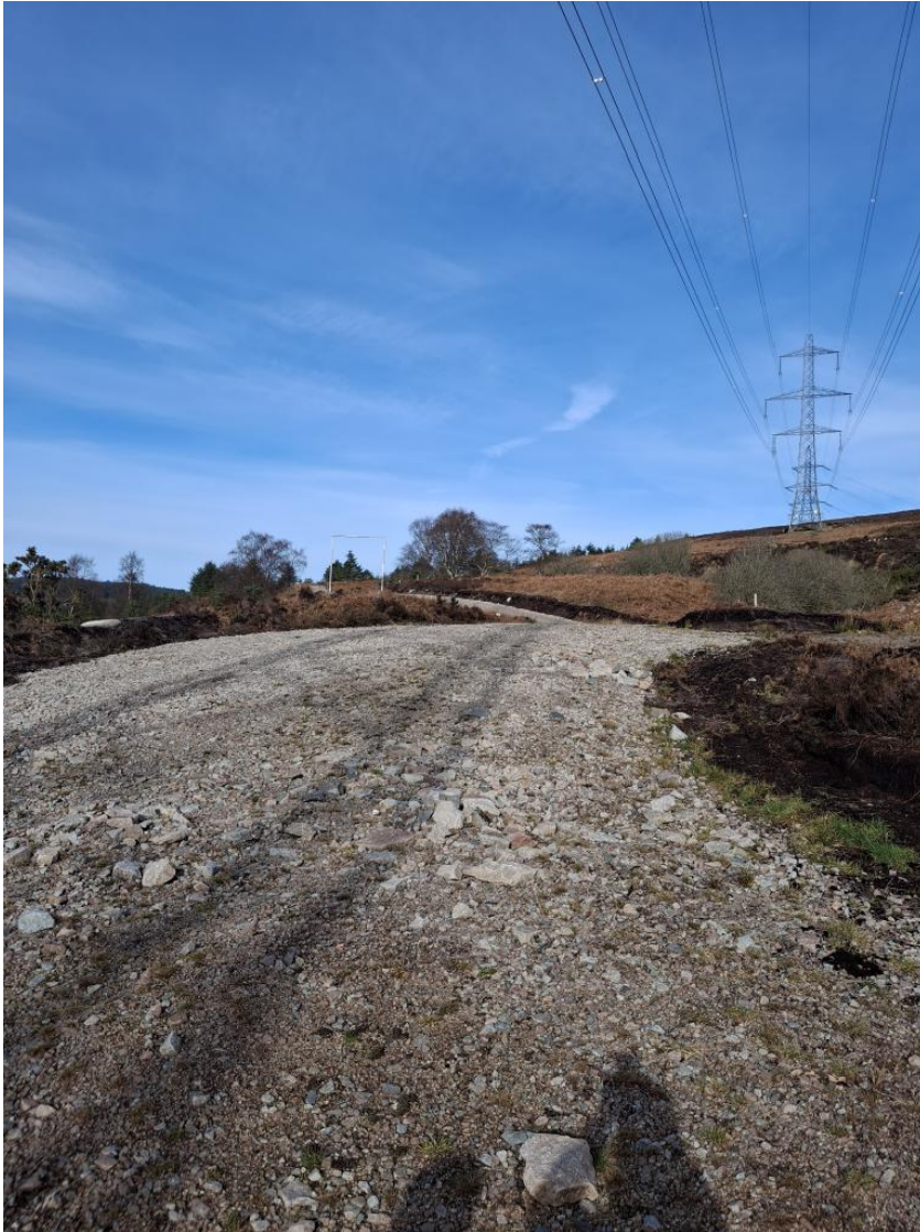
Plate 1: Looking north towards Tower N85
