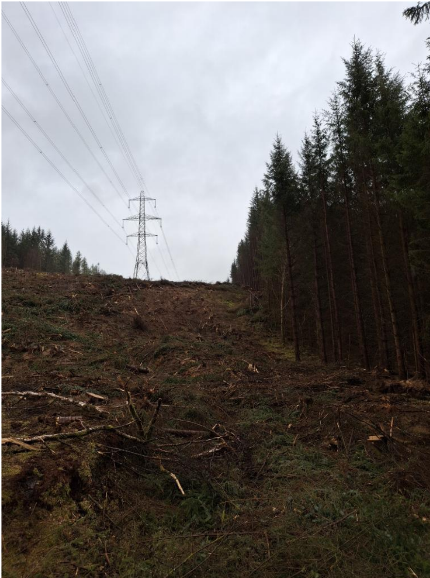
Plate 2: Looking south towards Tower N90
