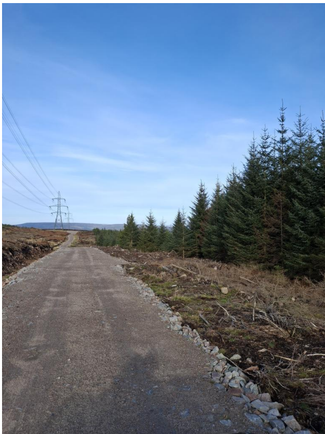
Plate 1: View from Tower N74 towards N73 facing NW.
