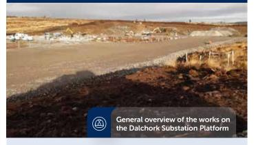
The works to A836 public road has been completed with traffic management removed at the beginning of October 2020. The platform construction is nearing completion, with the blasting of rock for stone production completed in mid-November 2020. Rock processing is ongoing to generate materials for platform construction.
