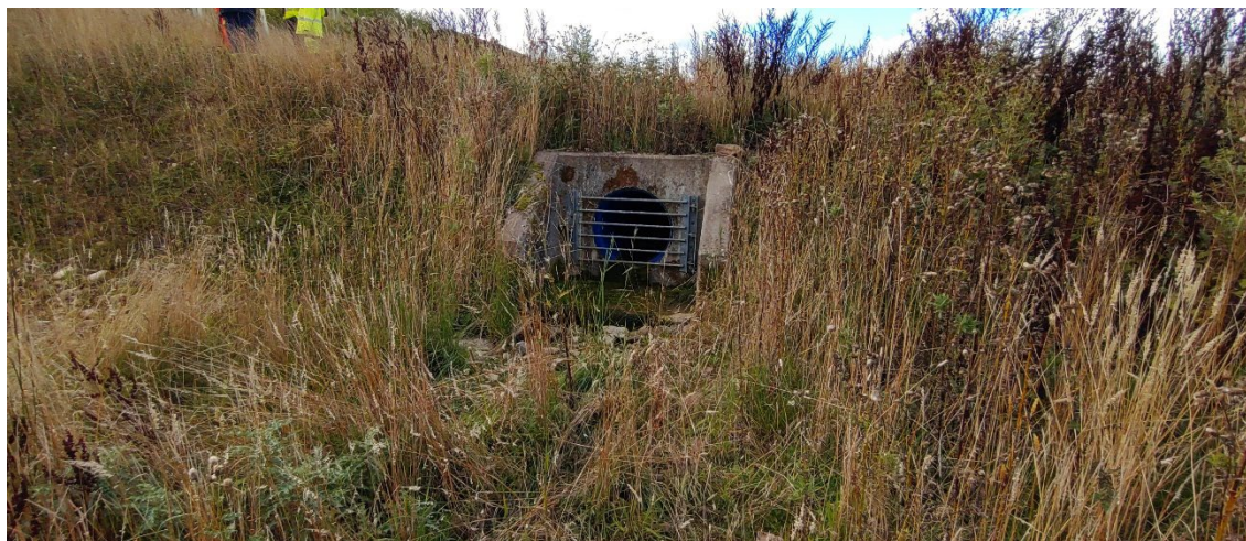
Figure 4.5: Existing Detention Basin Headwall
