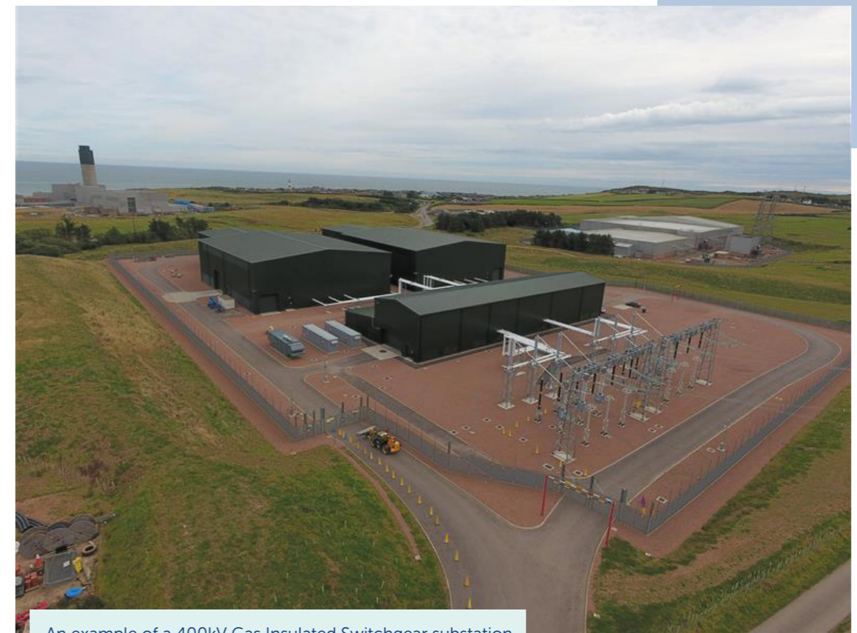
An example of a 400kV Gas Insulated Switchgear substation
