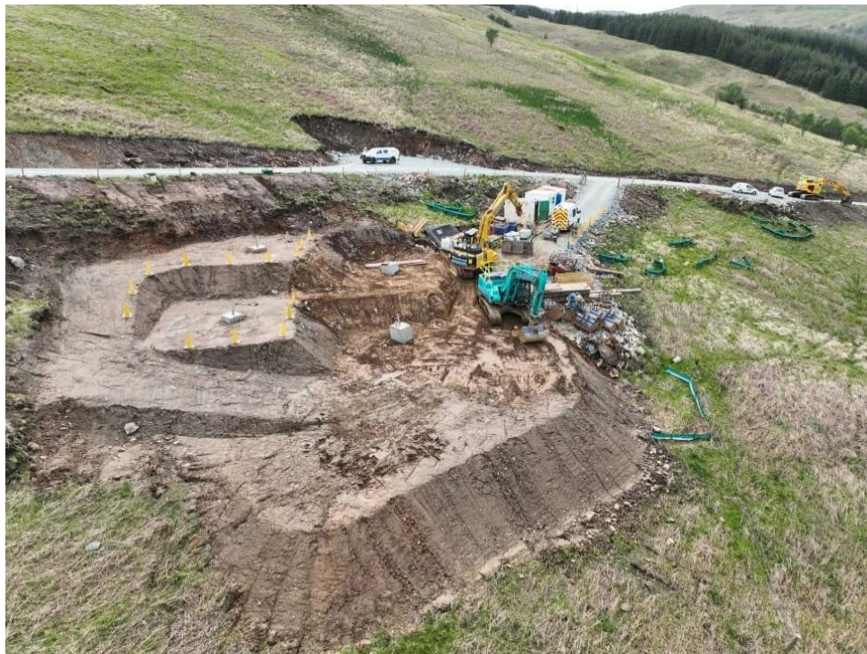
Plate 2.2: Illustrative Image of Tower Foundation Construction
