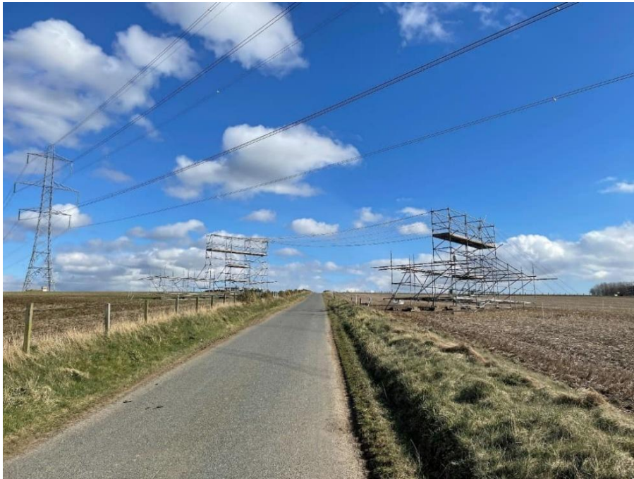
Plate 2.4: Illustrative Image of Temporary Construction Scaffolds
