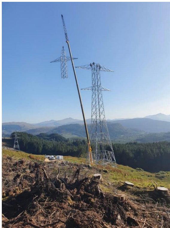
Plate 2.3: Illustrative Image of Tower Construction
