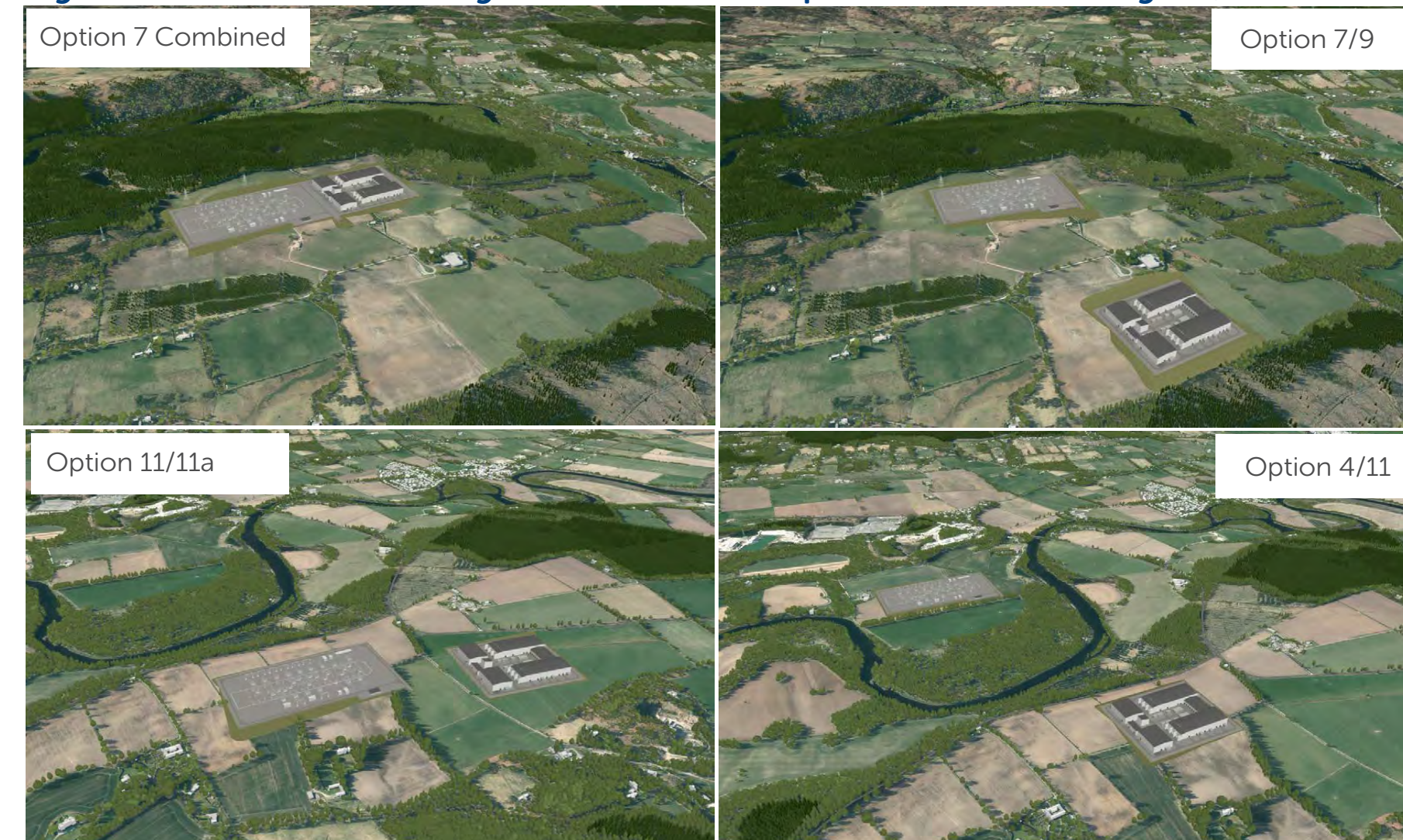
Figure 8: Indicative Aerial images of the Four Site Options Assessed at Stage 2 (Detailed Site Selection)
