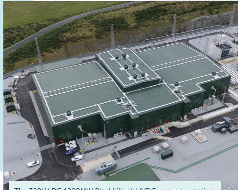
The 320kV DC 1200MW Blackhillock HVDC converter station
