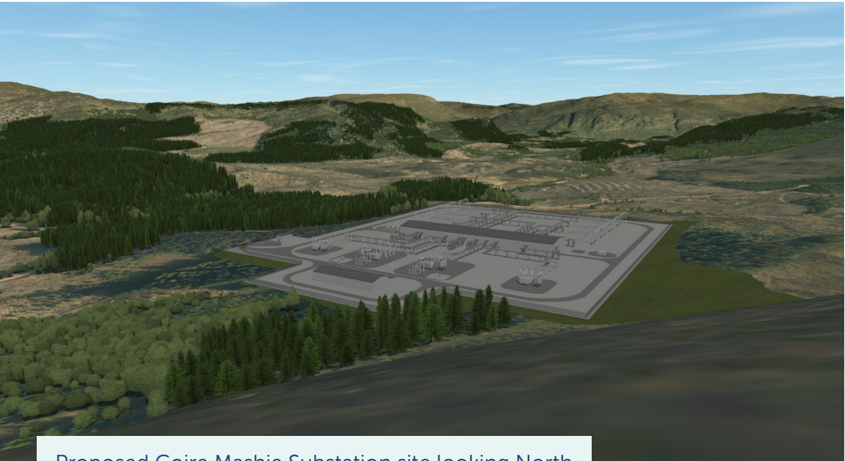
Proposed Coire Mashie Substation site looking North
