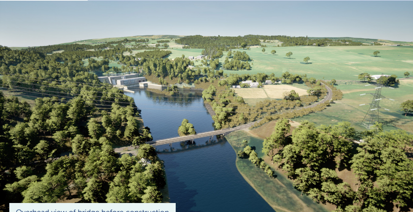
Overhead view of bridge before construction
