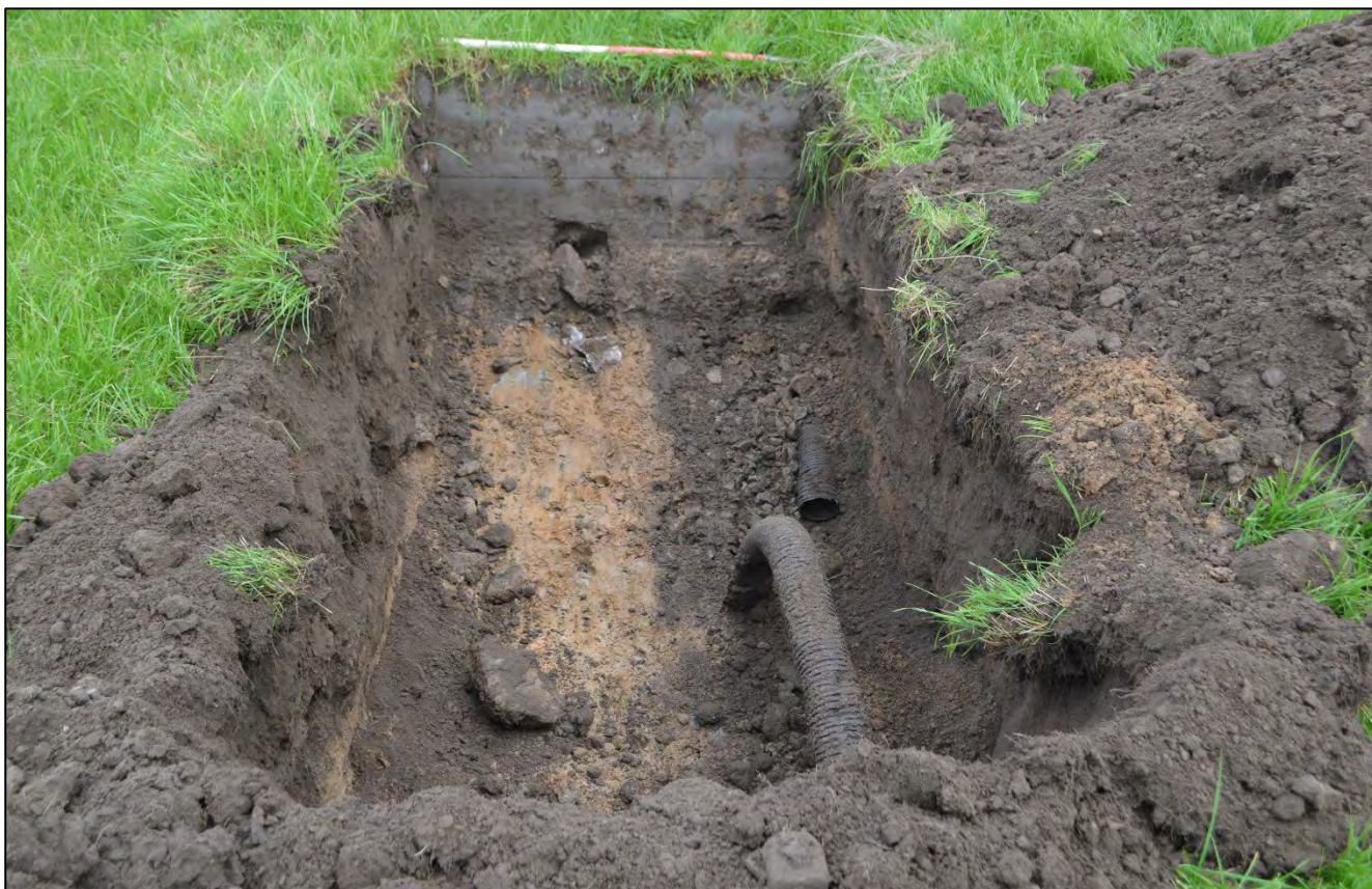
Plate 2: Example of field drain requiring new Test pit location
