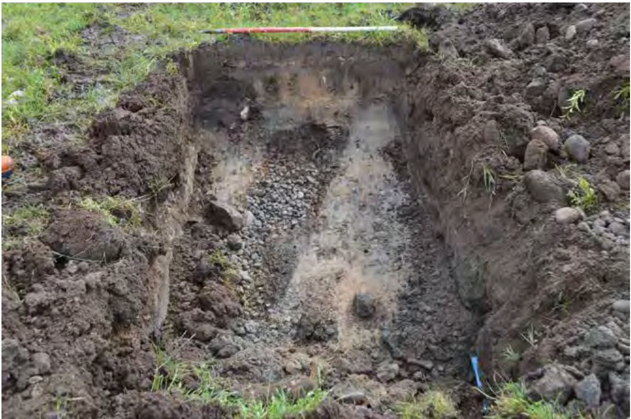
Plate 93 Post-excavation of TP72, including location of field drain and blue water service pipe
