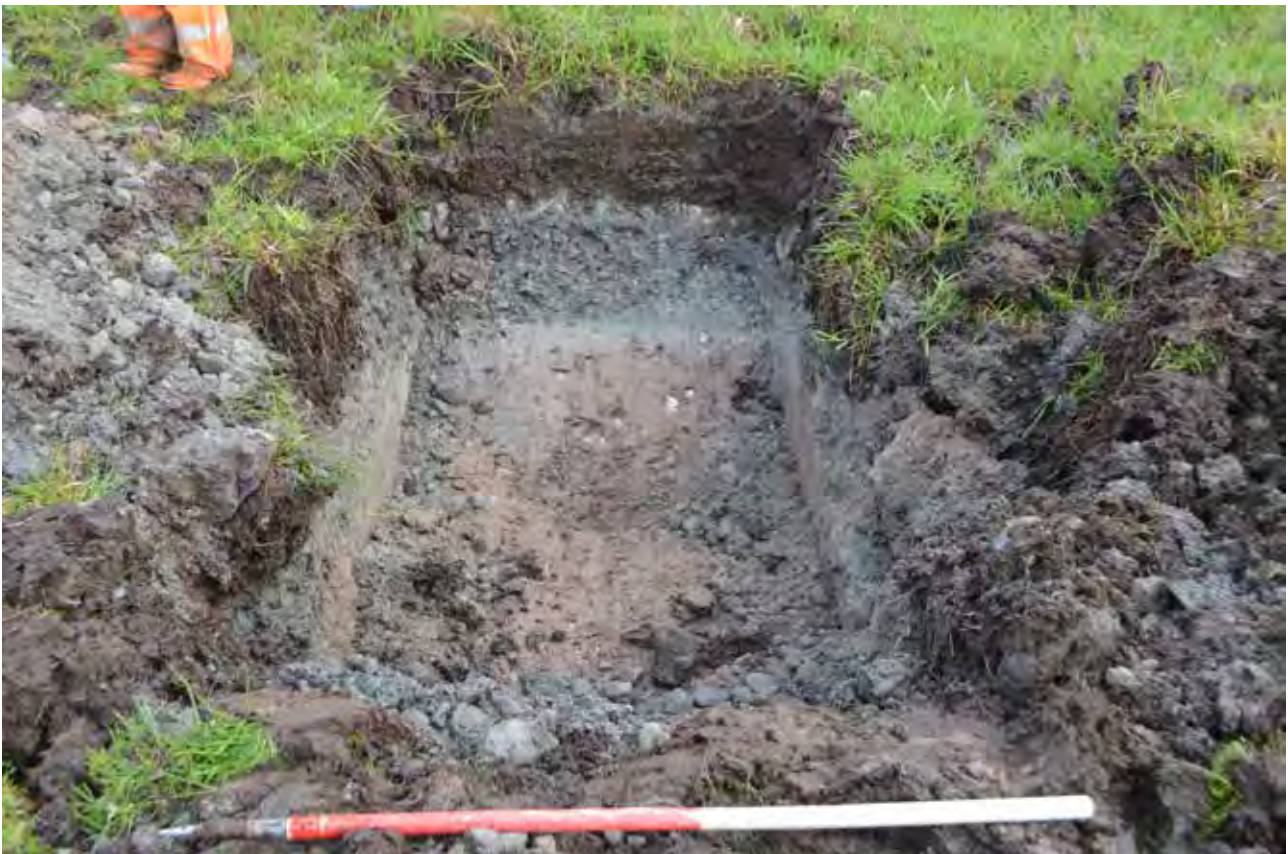
Plate 85 Post-excavation of TP65 showing topsoil over clay layer
