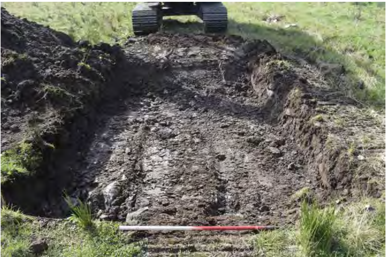
Plate 11 Post-excavation of TP4.1 extended for plate load test
